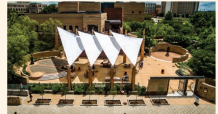
Rear exterior view of the Eiteljorg Museum, showing The Sails, an outdoor shade structure under which music and dance performances are held, and the Christel DeHaan Family Terrace Image courtesy of Zach Malmgren
